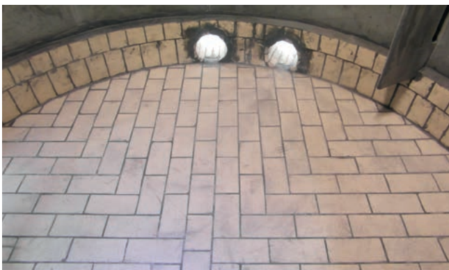
Brick lining a tank floor with Furan Mortar
