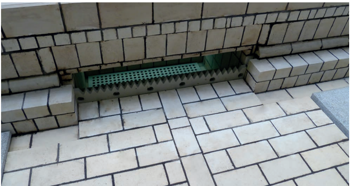
Brick lining with Furan Mortar.
